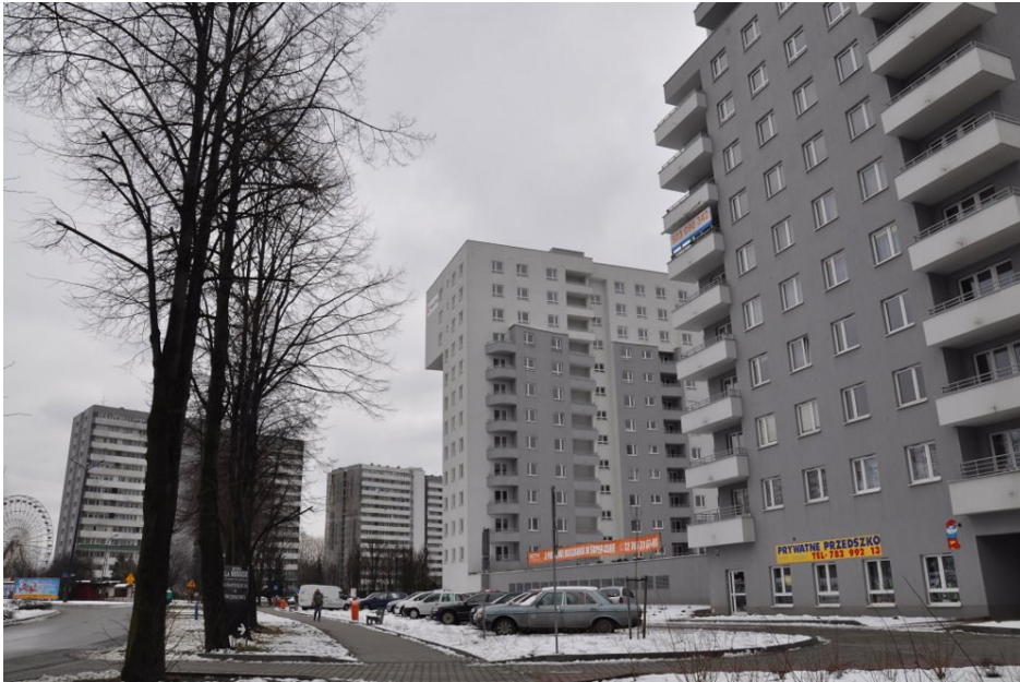
Picture 22. Katowice, Tysiąclecie estate (built in the 1960s and 1970s): new multi store apartment buildings (from 2010) with 160 flats (39m 2 -140m 2 ). Price started at 4500 PLN for 1m 2 in 2010. Photo: A.Cieśla, 2011
