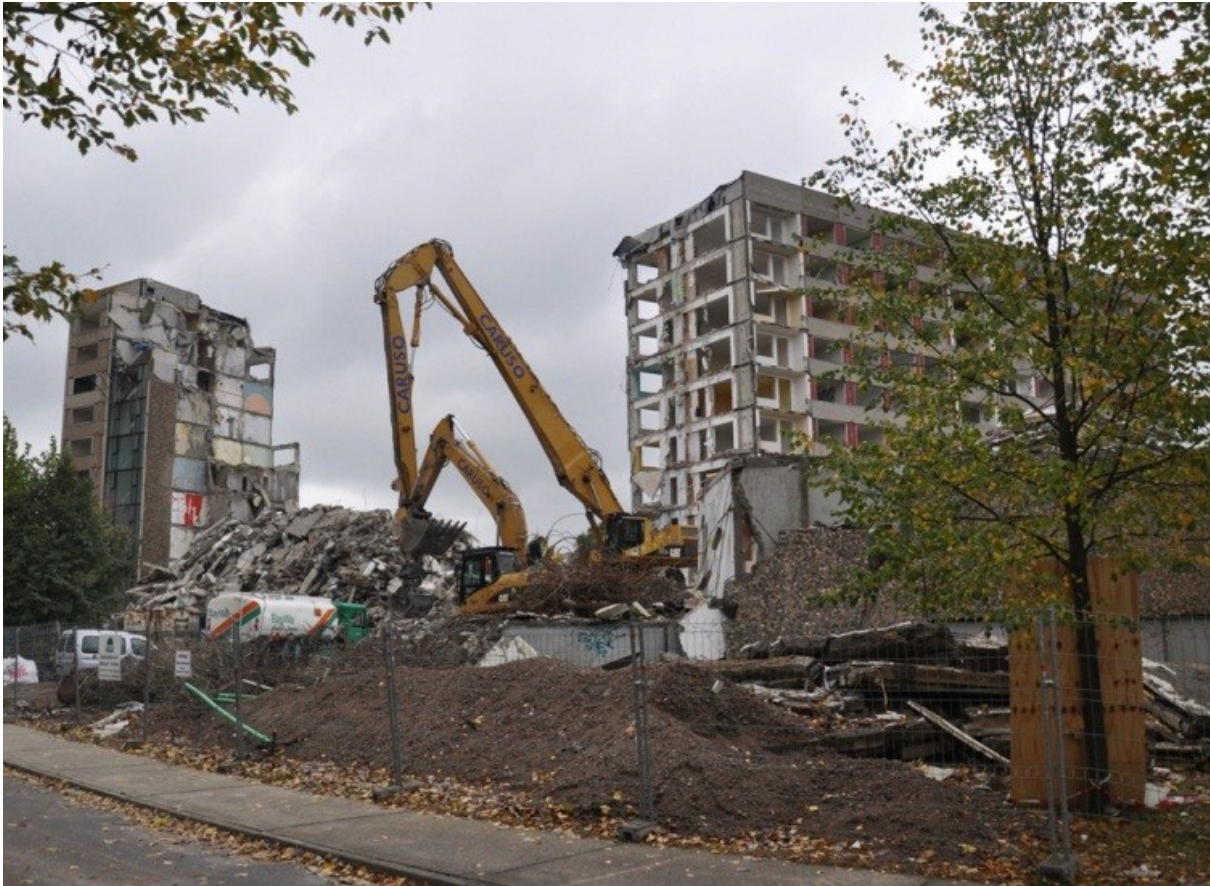
Picture 14. Perforating urban structure in Eastern Germany. Demolition of prefabricated buildings in Dresden, March 2010, photo: Ciesla
