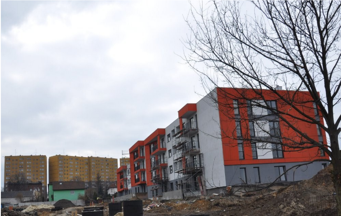
Picture 24. Gliwice, Kozielska Street: new multi store apartment building with 51 flats (27m 2 -75m 2 ), investment finished in April 2011. Price: 4940PLN-5463PLN for 1m 2 , photo: A.Cieřla, 2011
